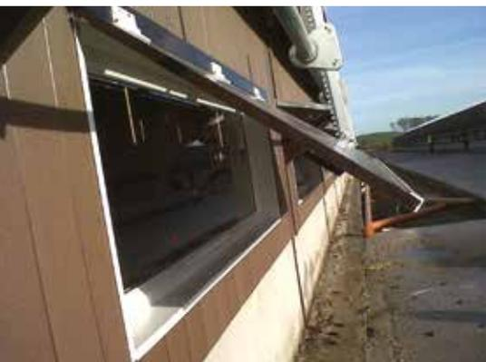
**A rack and pinion shutter system on a broiler shed**
